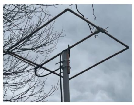
Construction was really easy with the ½" copper and various other parts being sourced at Menard's. The design and plans were pulled off the internet, so that was pretty easy. The bill of materials is below. Everything except the coax and SO-239 is literally falling off the shelf.
