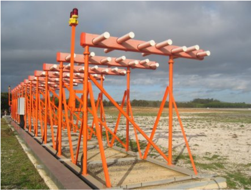
ILS (Instrument landing system) Localizer Antenna system. Provides horizontal alignment on runway.
