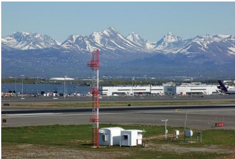
Above: ILS glide slope antenna system provides vertical glide path to runway. Normally 3 degrees.
